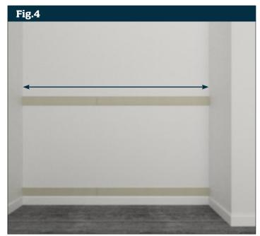
Measure distance between top and bottom strips and cut 4 vertical panel strips. Apply adhesive to back of strips. Offer 2 strips between horizontal strips, placing one of them at each end of the run. Secure with nail gun **(Fig 5)**.
