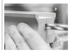
Cut the handrail to the correct angle & length. Position against newel post and mark the height on the newel (from the underside of the handrail).
