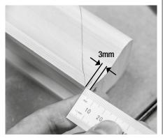
Mark the centreline of the handrail 24mm up from the base. (Including the infill strip).
